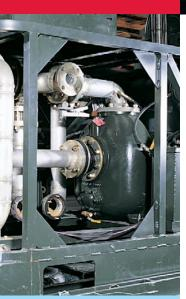
Gorman-Rupp O Series® self-priming centrifugal pumps have a straight-in suction design which eliminates entrance restrictions and provides better performance when handling a variety of clear liquids.
